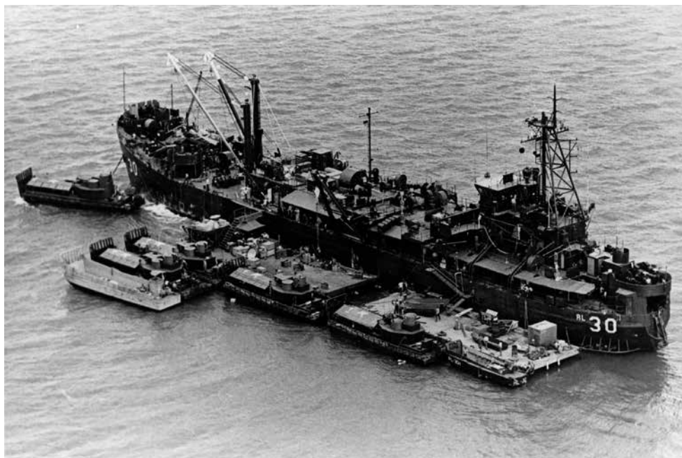
One of the three mobile bases for the Mobile Riverine Force, the landing craft repair ship Askari (ARL-30) provides maintenance and support for various craft assigned to the command, May 1967.
